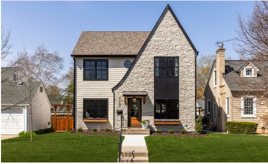
Entire House $750,000 to $1,000,000 (Gold) Anchor Builders
